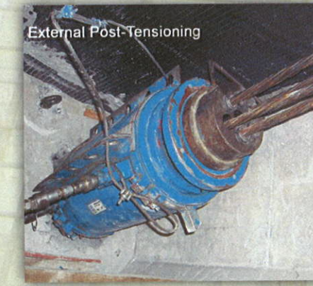
LTA Contract RD222 Upgrading of Vehicular Bridges at 5 Locations Includes External Post-tensioning
