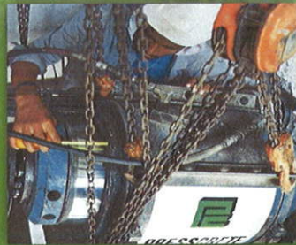
Post-Tensioning Using Multi Strand Jacks
