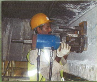
Stress Bars Tensioning
